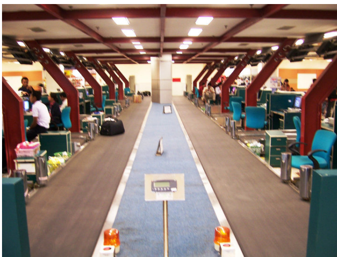
The check-in conveyor end-up at the heavy duty collecting conveyor
