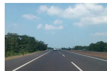
Good pavement in Cipali Highway, West Java, MBW's partner in progress
