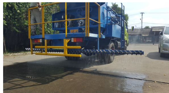
Spraying in test
